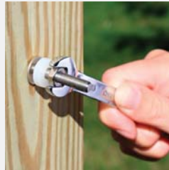
Step 1 Tighten nut to tension.
