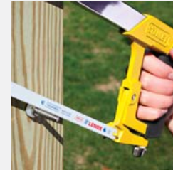
Step 2 Cut thread flush with nut.
